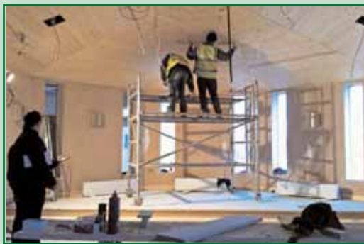
Worship area in progress
